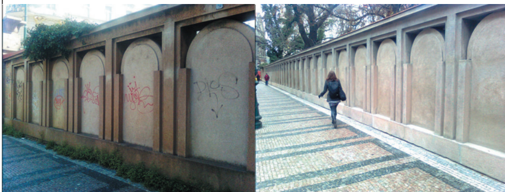
The walls of the Old Jewish Cemetery before and after repairs
