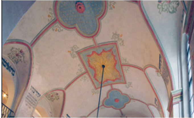
Stucco and painted decoration on the arch in the Rear Synagogue in Třebíč after renovation
