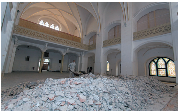
Demolition of the modern floor in the Maisel Synagogue
