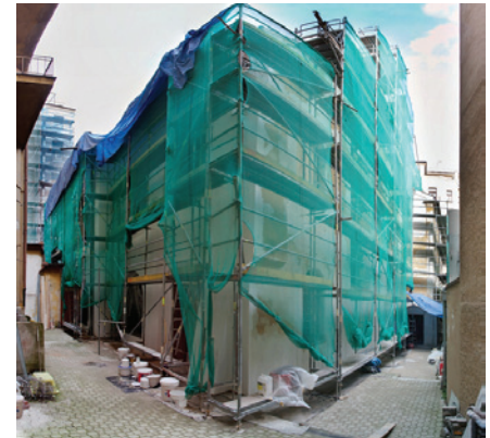
Repairs to the outside walls of the Maisel Synagogue.
