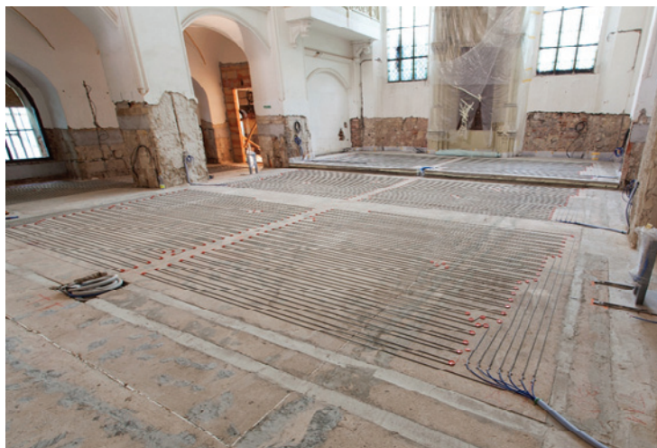
Work on the underfloor cables in the Maisel Synagogue.
